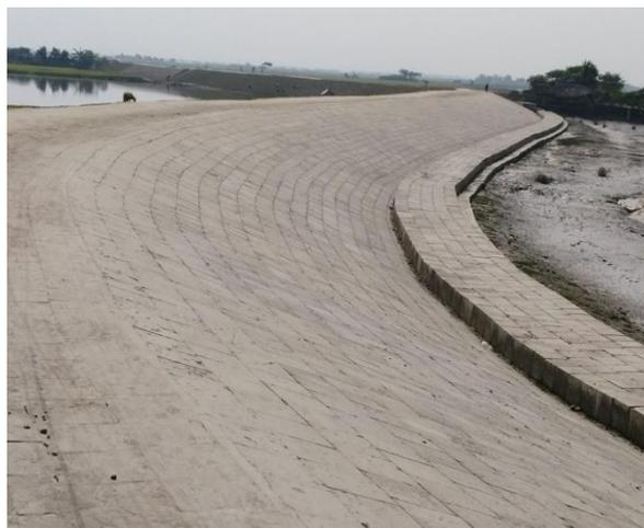
Figure 3-34: Completed Slope Protection Works in Polder-32
