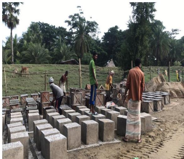
Figure 3-63: CC block manufacturing in Polder 47/2 at yard-1
