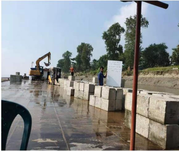
Figure 3-58: Dumping work in Polder-41/1
