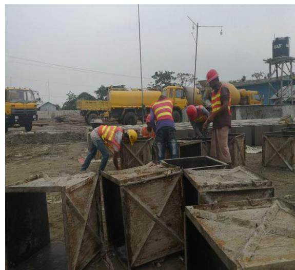
Figure 3-67: CC Block Manufacturing at Yard 1 in Polder 48
