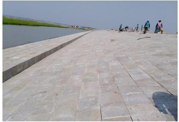
Figure 3-38: Completed Slope Protection Works in Polder-32
