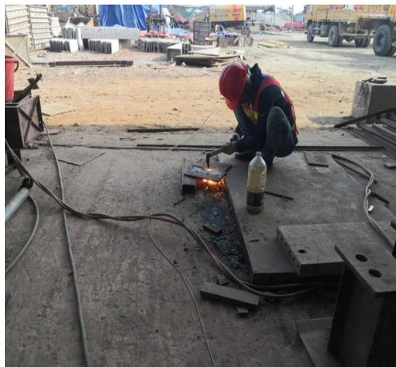
Figure 3-65: Repair formwork for CC block in Polder 48
