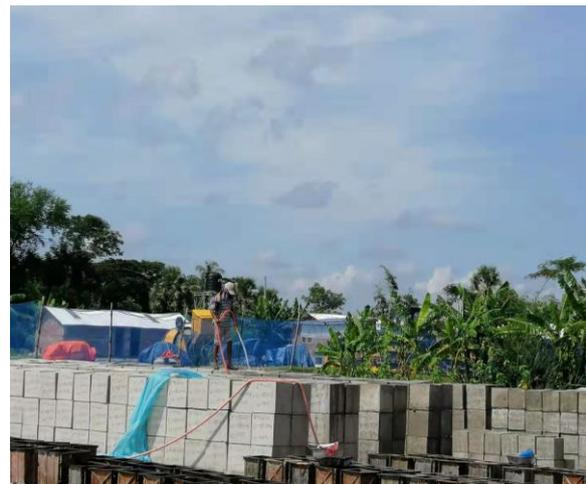
Figure 3-61: Curing CC Blocks in Polder 43/2C at DS-1 yard
